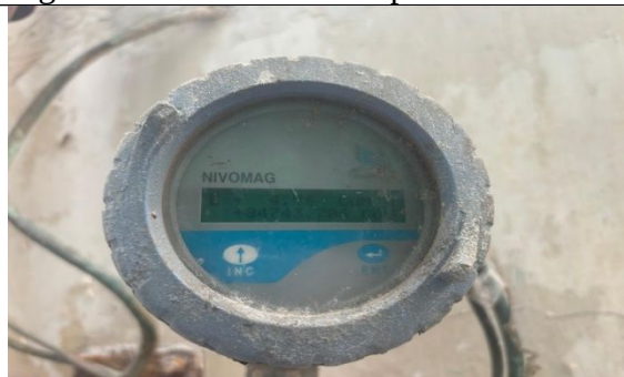
Figure 1: Magnetic Flow meter at borewell
